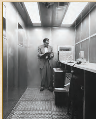
Figure 3 Willis Whitfield in prototype "laminar flow" cleanroom. 13
