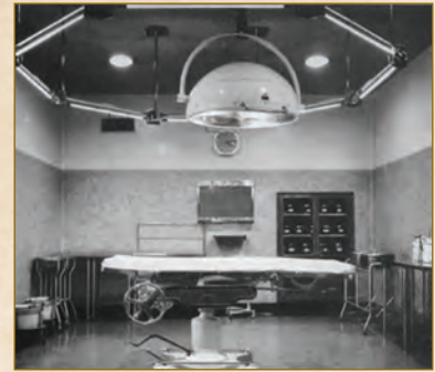
Figure 1 1936 Operating room showing UV lamps. Air inlet in the upper left. 7
