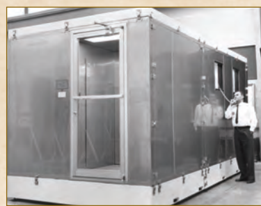
Figure 4 Willis Whitfield's "knock-down" portable cleanroom. 13
